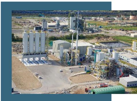
Applying this technology, the P2O5 in rock phosphate is gently dissolved in dilute acid to obtain a dilute solution of phosphoric acid and monocalcium phosphate (MCP). The liquid solution is further purified to reduce the level of heavy metals to far below EU requirements. Calcium carbonate (CaCO<sub>3</sub>) is then added to precipitate out a very pure dihydrate dicalcium phosphate. In the final stage, this precipitate is granulated and dried.
