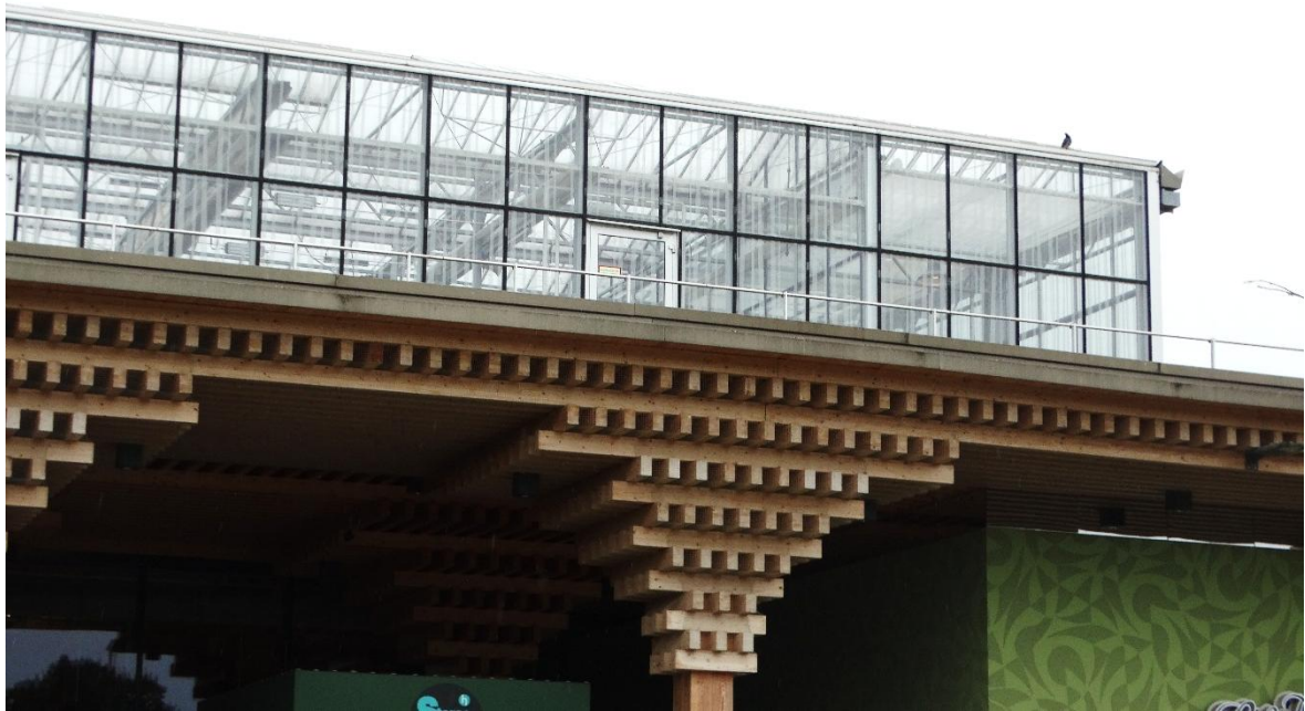
Abbildung 15: Green Building REWE Wiesbaden-Erbenheim
